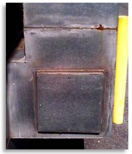
This duct access panel should be fully attached and the corrosion checked for potential failure points.
