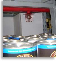
This pendent sprinkler with a shield installed in rack storage is one special sprinkler example. The shield at the top is to help prevent the sprinklers from being wetted (cold soldered) from water spray of higher elevation sprinklers.
