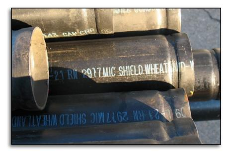
Photo courtesy of Freedom Fire Protection, LLC, Longmont, Colorado. This treated ferrous pipe may not be compatible with chlorinated polyvinyl chloride
